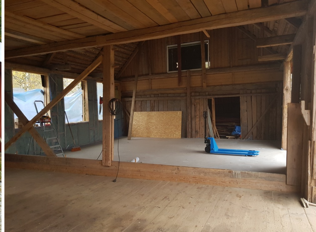
Concrete floor and back walls in place, windows delayed
